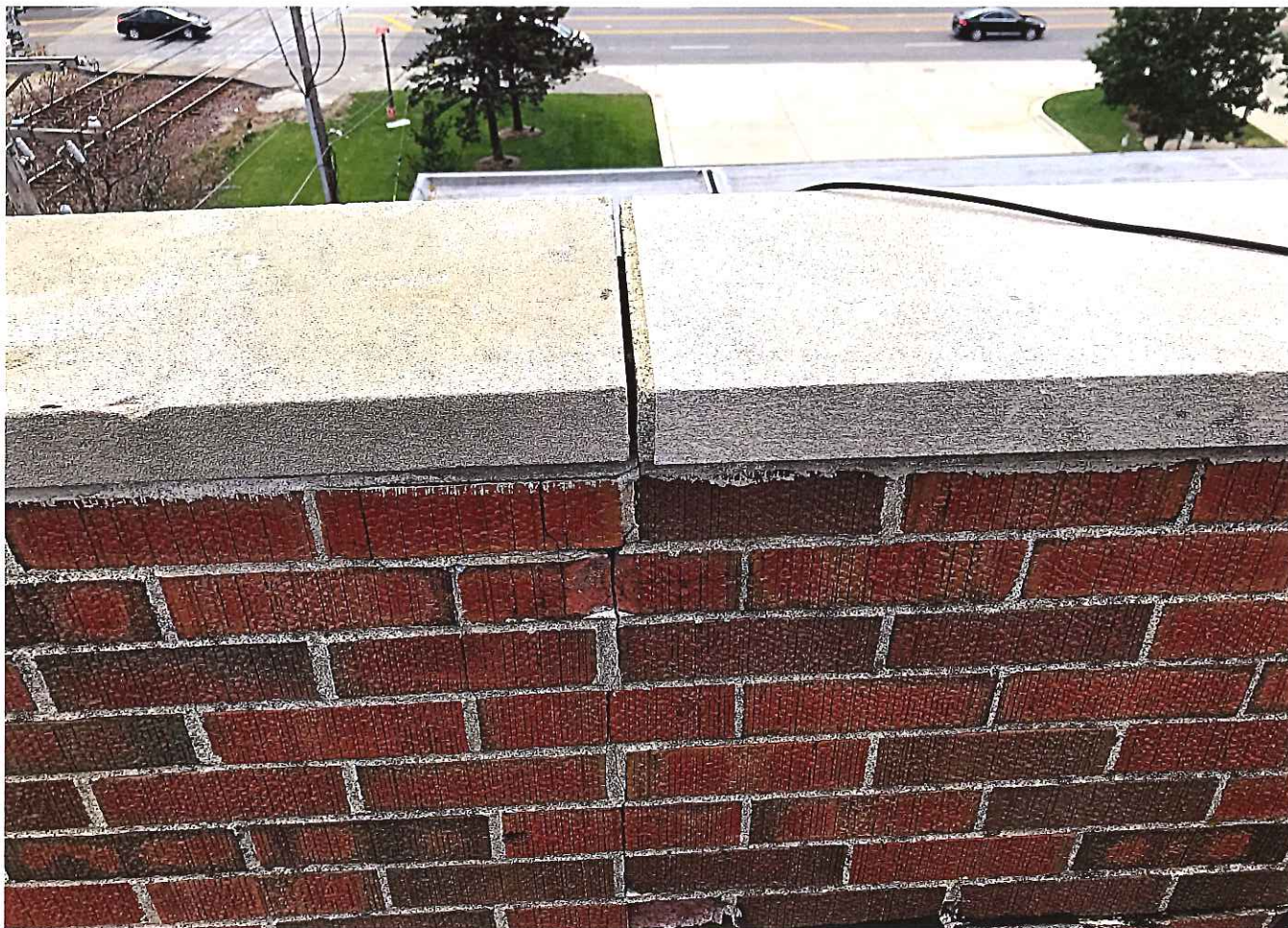
(ST-5) Masonry deterioration
