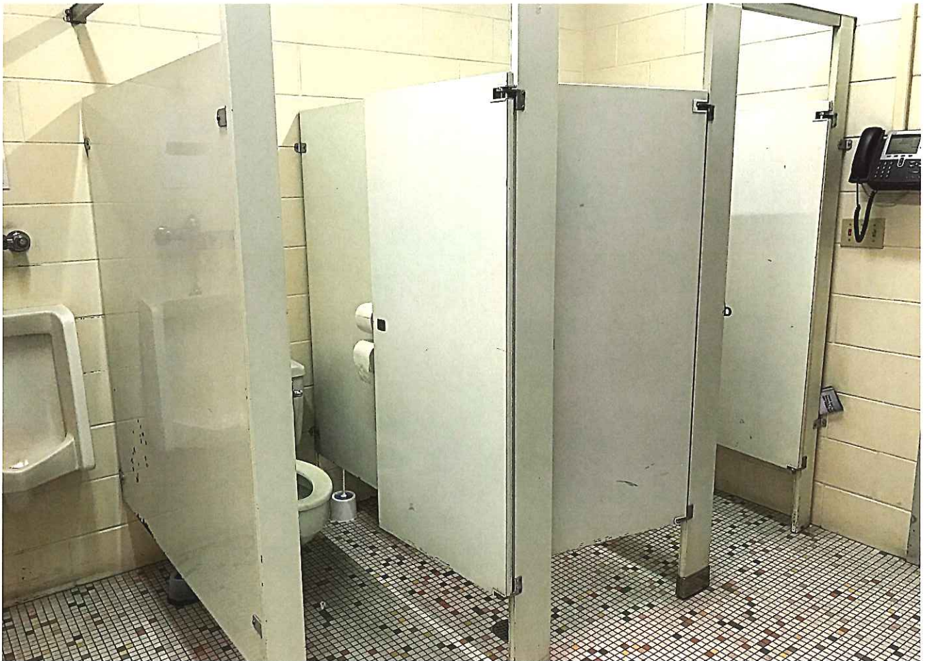
(BE-6 & A-6) No accessible toilet facilities or female toilet facilities - Finishes are worn
