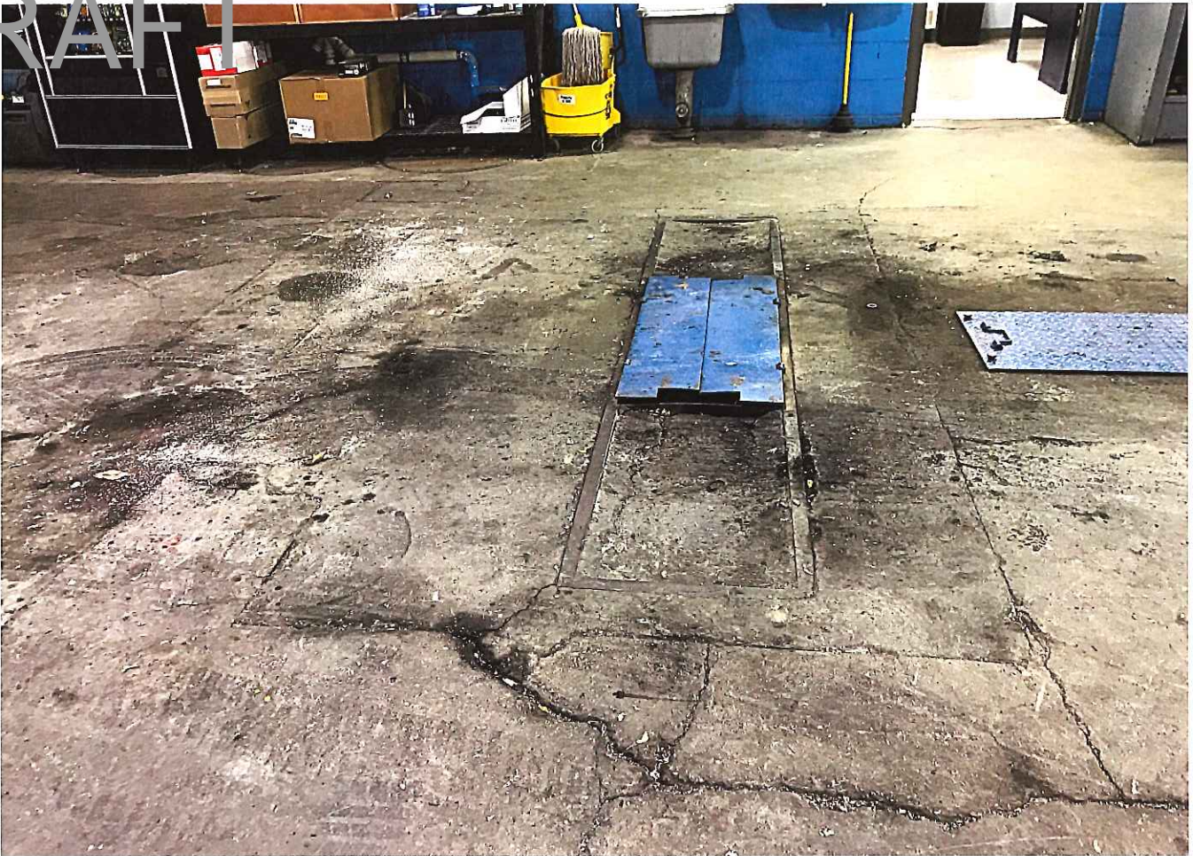
(ST-1) Pitting and Spalling concrete
