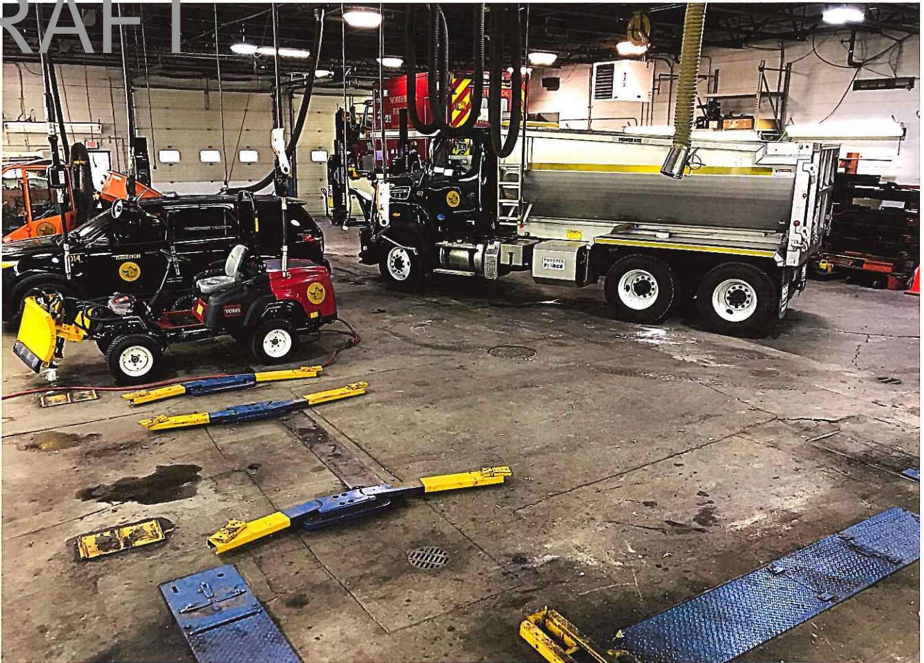
(A-8) Deteriorated concrete slabs and lifts
