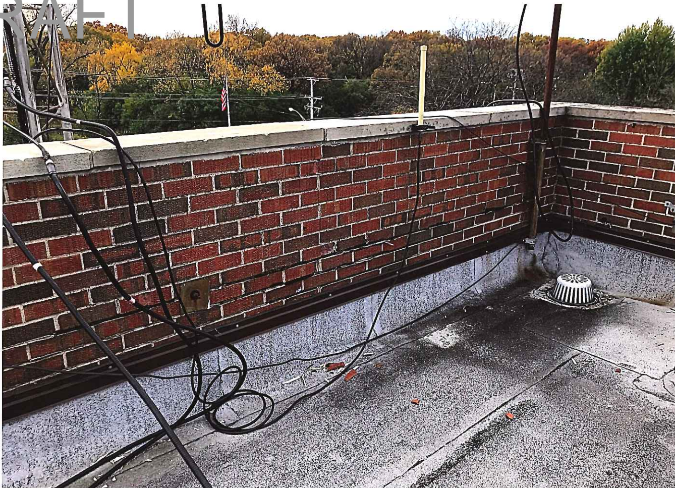
(ST-5) Masonry deterioration
