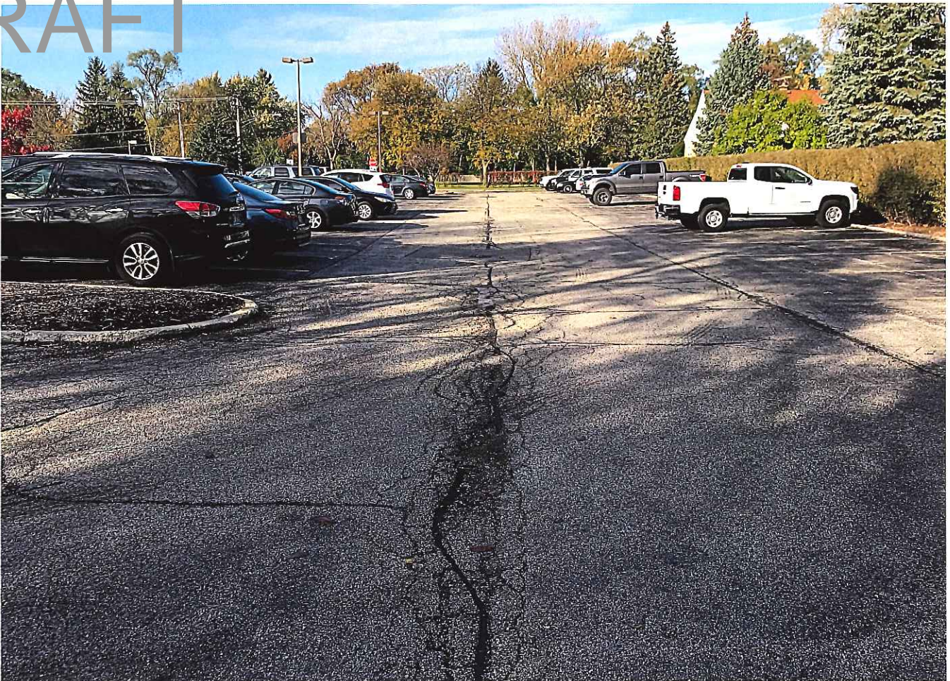
(S-4) Deteriorated parking lot paving
