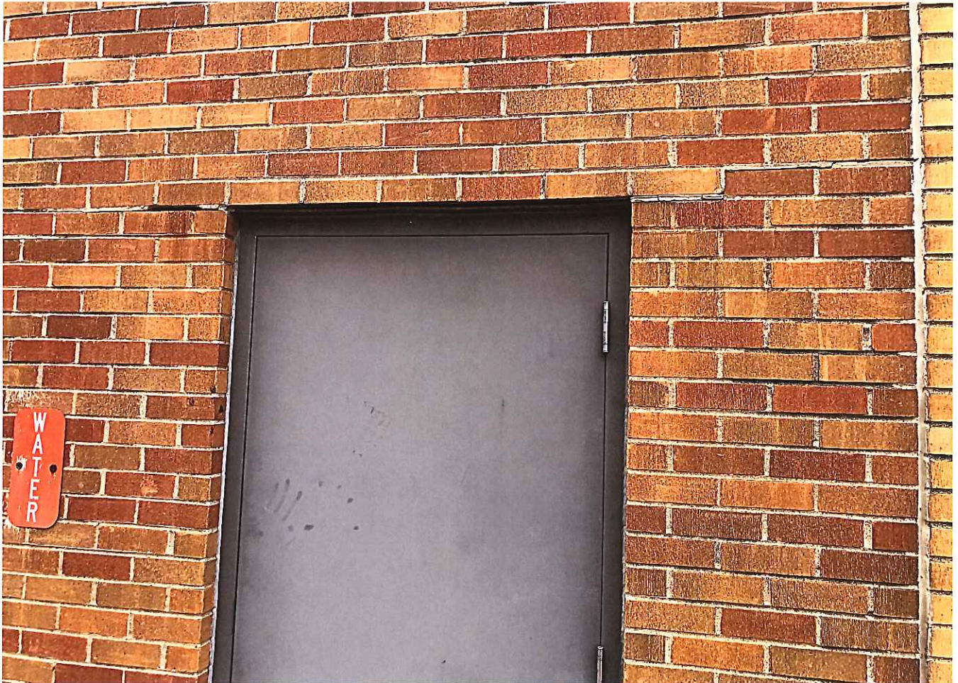
(A-3) Steel lintel is rust jacking
