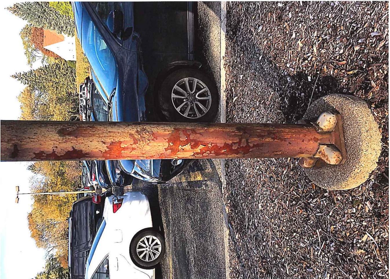
(S-4) Deteriorated site lighting poles
