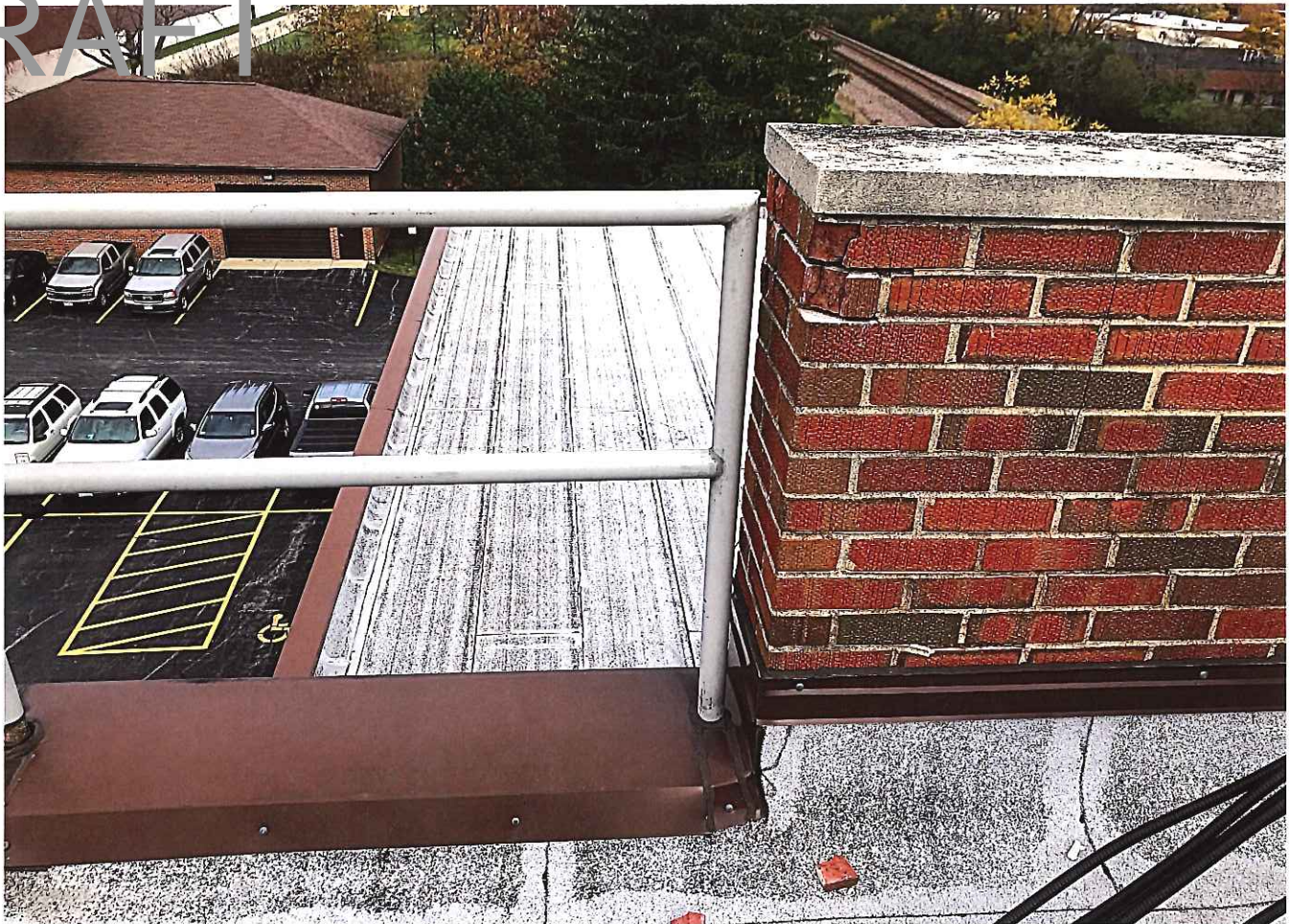
(ST-5) Masonry deterioration
