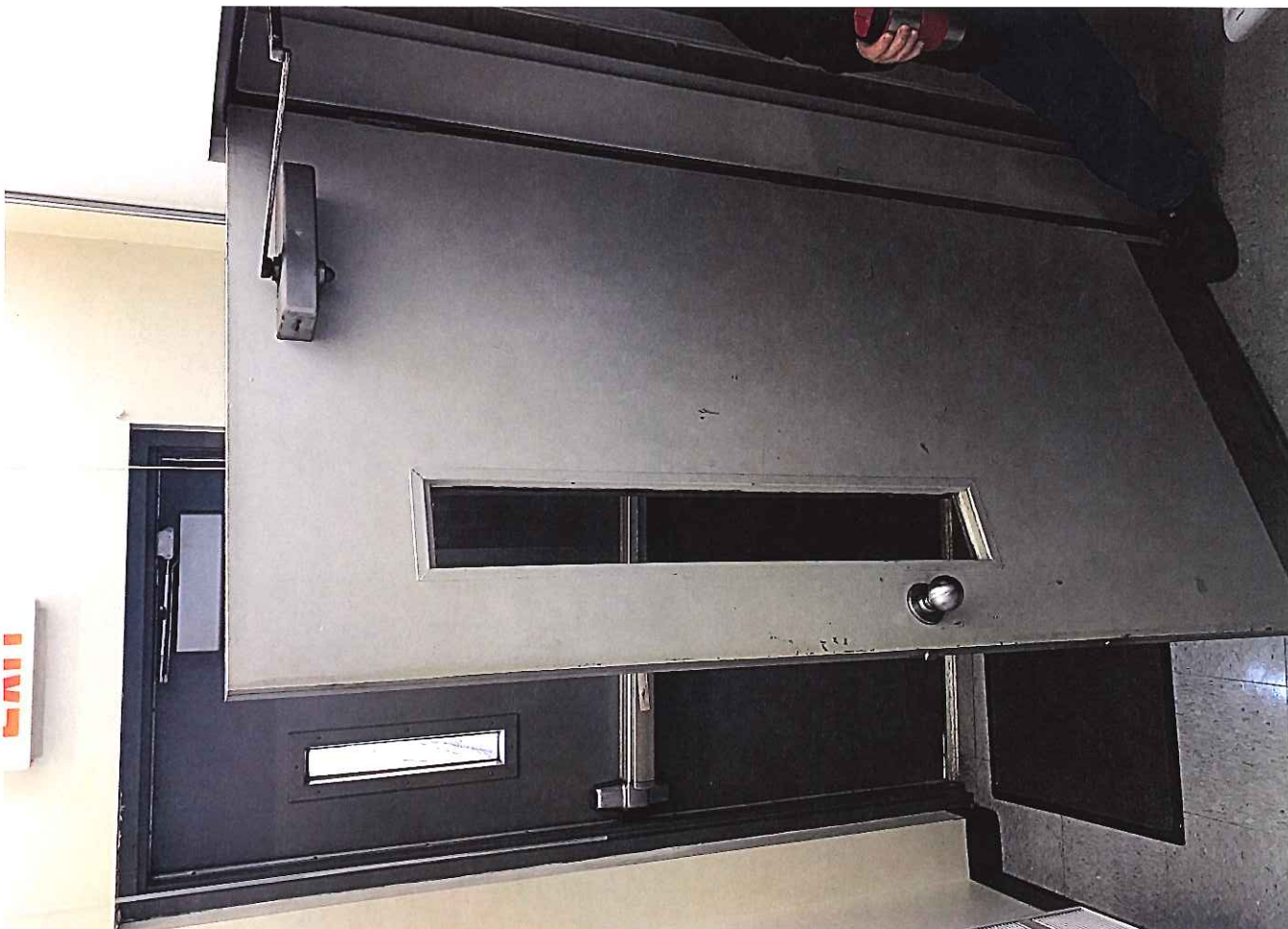
(BE-2) Exit door impedes egress through exit stair
