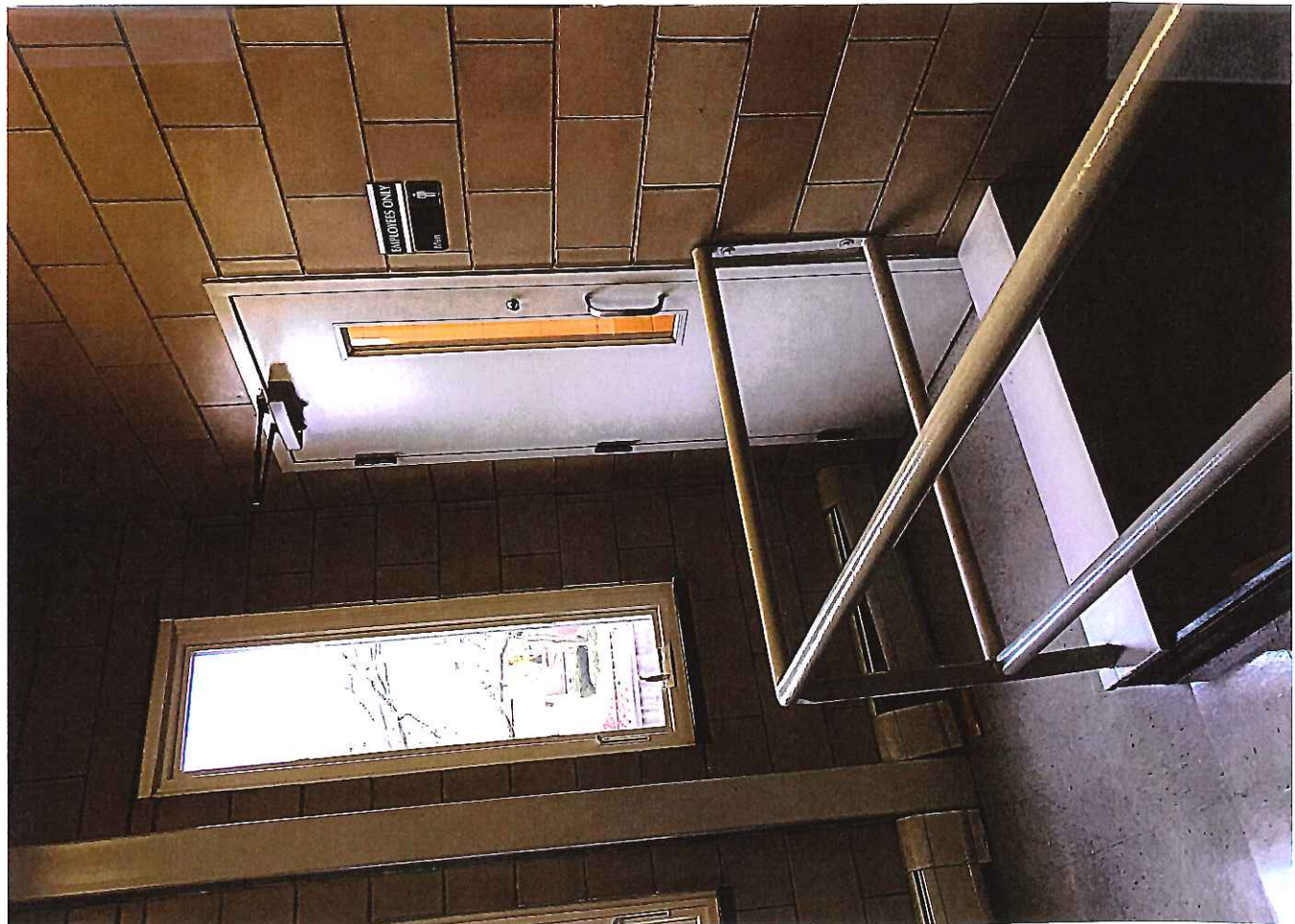
(BE-1) Missing door push/pull accessibility clearances
