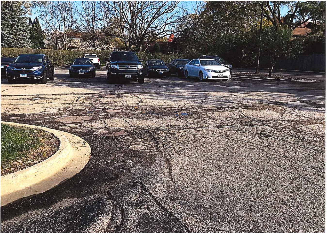
(S-4) Deteriorated parking lot paving
