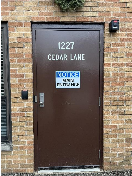
Access control at main entry door / Inaccessible door hardware
