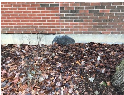
Previously patched foundation cracking at building addition
