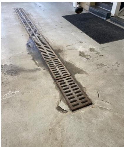
Concrete cracks and spalls at the apparatus bay slab on grade
