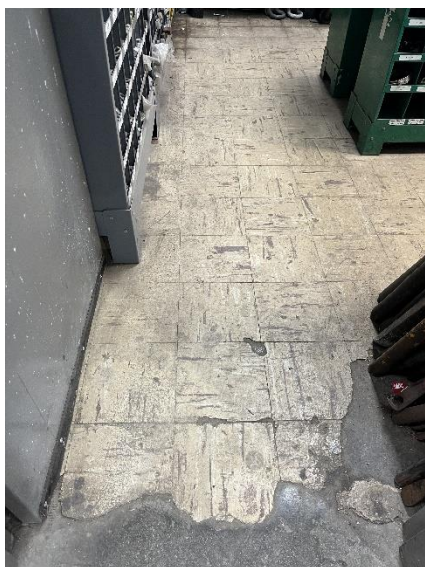
Suspected asbestos floor tile
