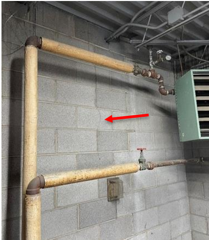
Thru-block crack at hose tower
