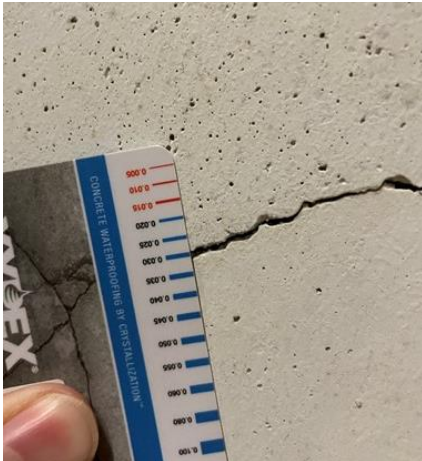
Minor concrete crack at basement wall
