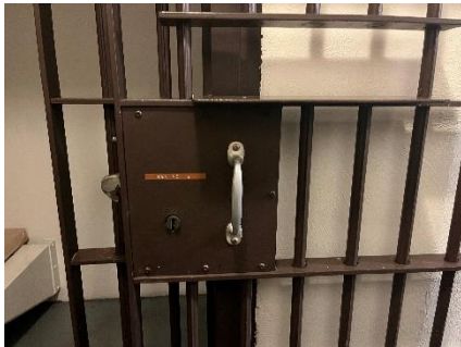
Cell doors are open steel bar fronts with manual locks
