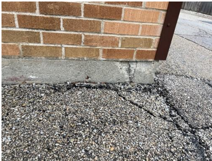
Cracks and spalls at exterior wall
