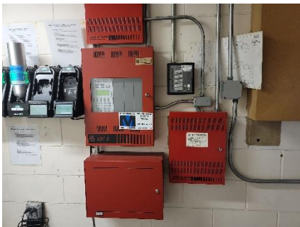
Fire alarm controls
