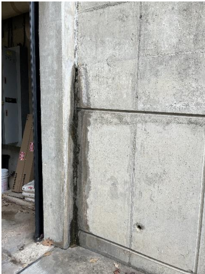
Seepage at concrete wall near exterior entry to garage
