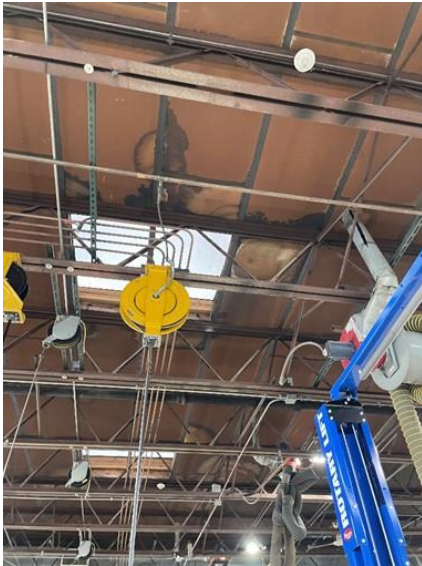
Significant water staining at skylight
