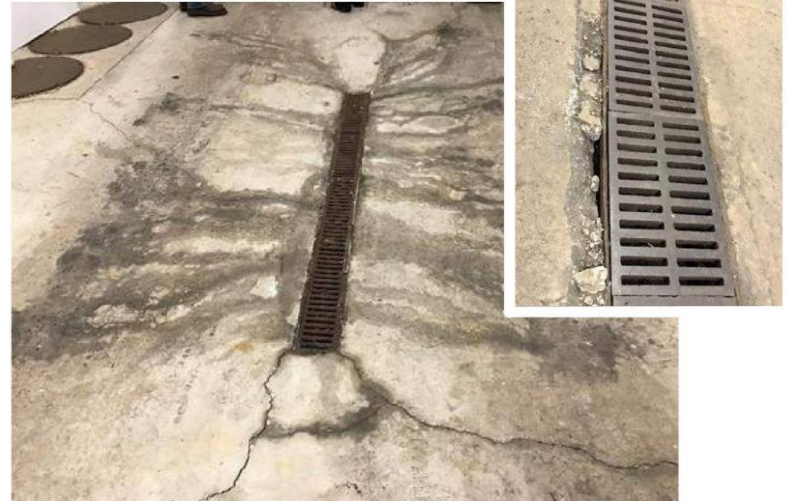
Concrete cracking at garage trench drain
