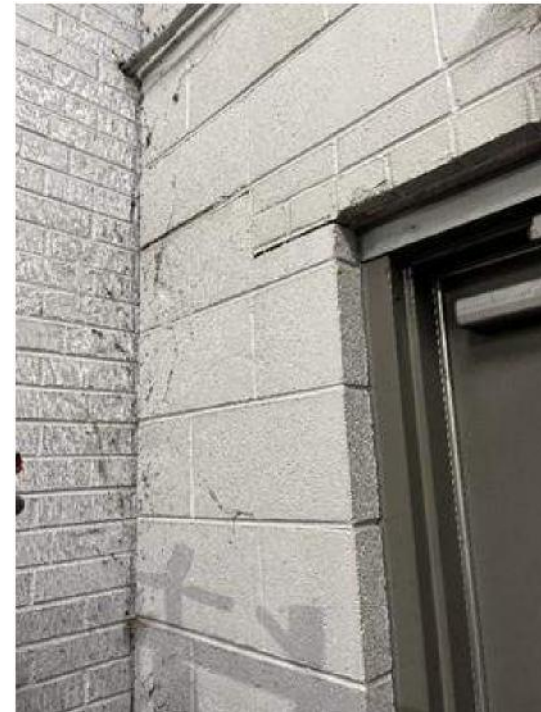
Step cracking at interior concrete masonry
