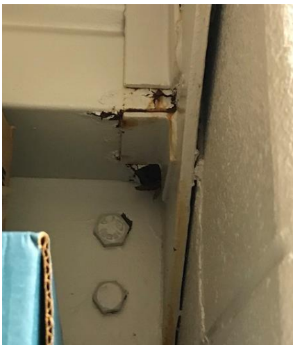
Corroded stair framing
