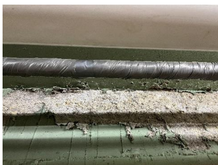
Deterioration at basement concrete wall
