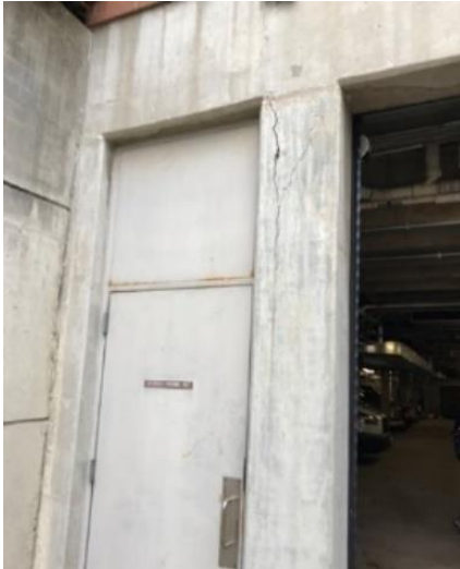
Column cracking adjacent to garage door
