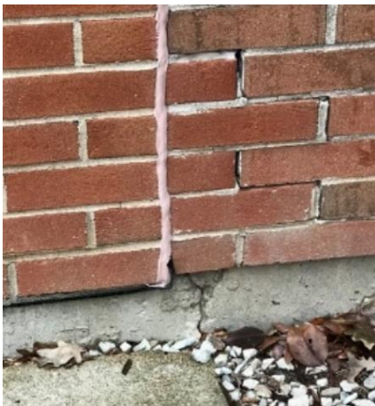
Foundation cracking at building addition
