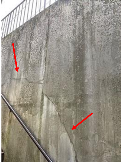
Significant concrete crack at basement stair
