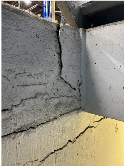
Cracking in concrete at stair to basement
