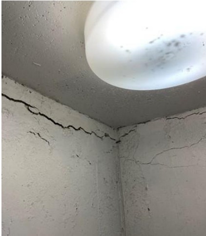
Concrete crack at basement stair
