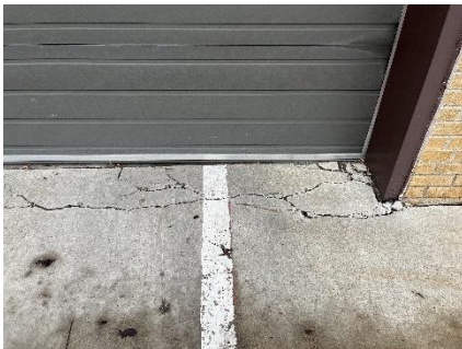
Cracking at overhead door concrete apron
