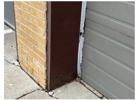
Deterioration of steel at overhead door jamb / broken door seals
