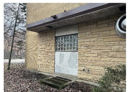
Typical deteriorated conditions at exterior wall and soffits
