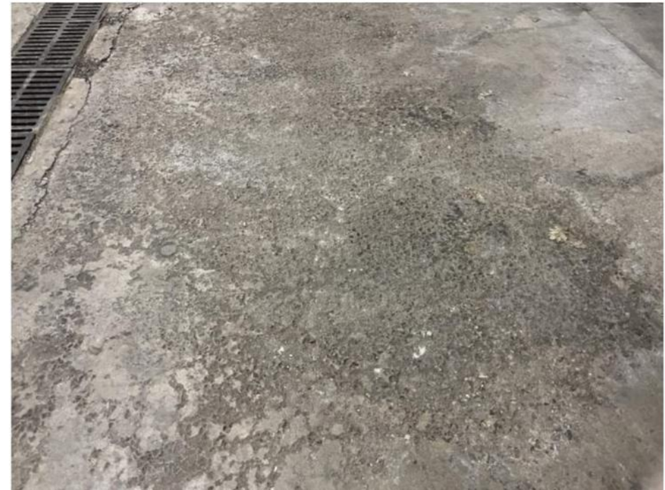
Deterioration in surface condition of concrete in garage
