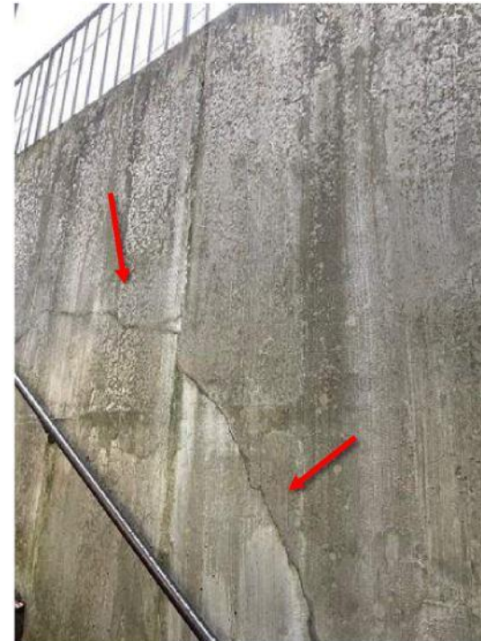
Significant concrete crack at basement stair
