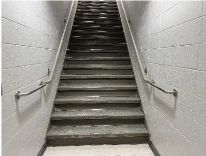
Retrofitted stair handrail extensions
