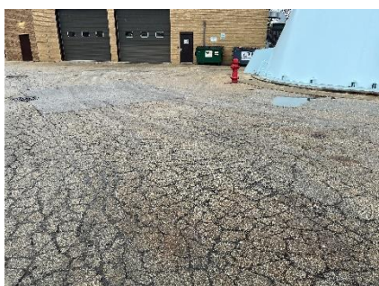
Cracking in asphalt pavement
