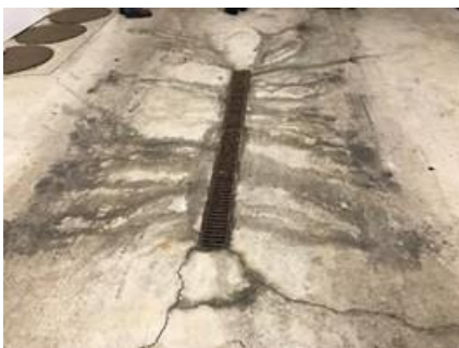
Concrete cracking at garage trench drain
