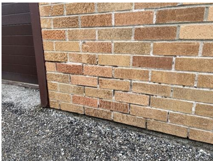
Missing / deteriorated mortar at exterior wall
