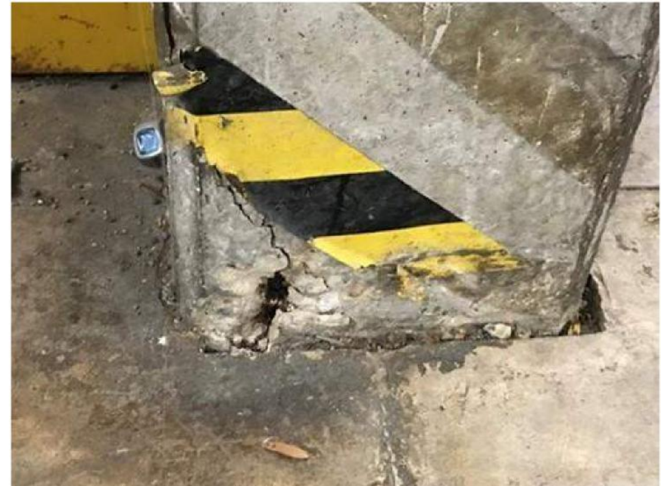
Column cracking at garage column
