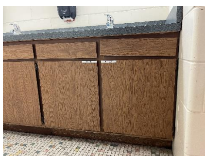
Deterioration at plastic laminate countertops and Interior cabinetry observed in numerous areas
