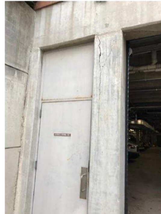
Column cracking adjacent to garage door
