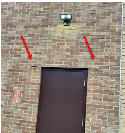
Step cracks and masonry displacement
