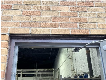
Displacement and gap at lintel
