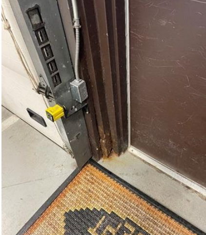
Significant corrosion at base of steel column in the Apparatus Bay
