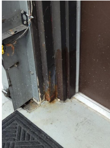
Significant corrosion at hollow metal door and frame
