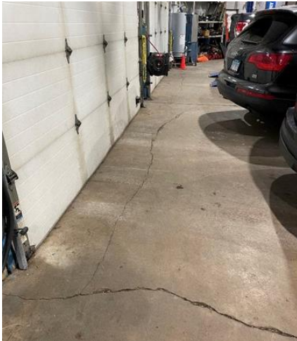
Global concrete cracks and spalls in the slab on grade
