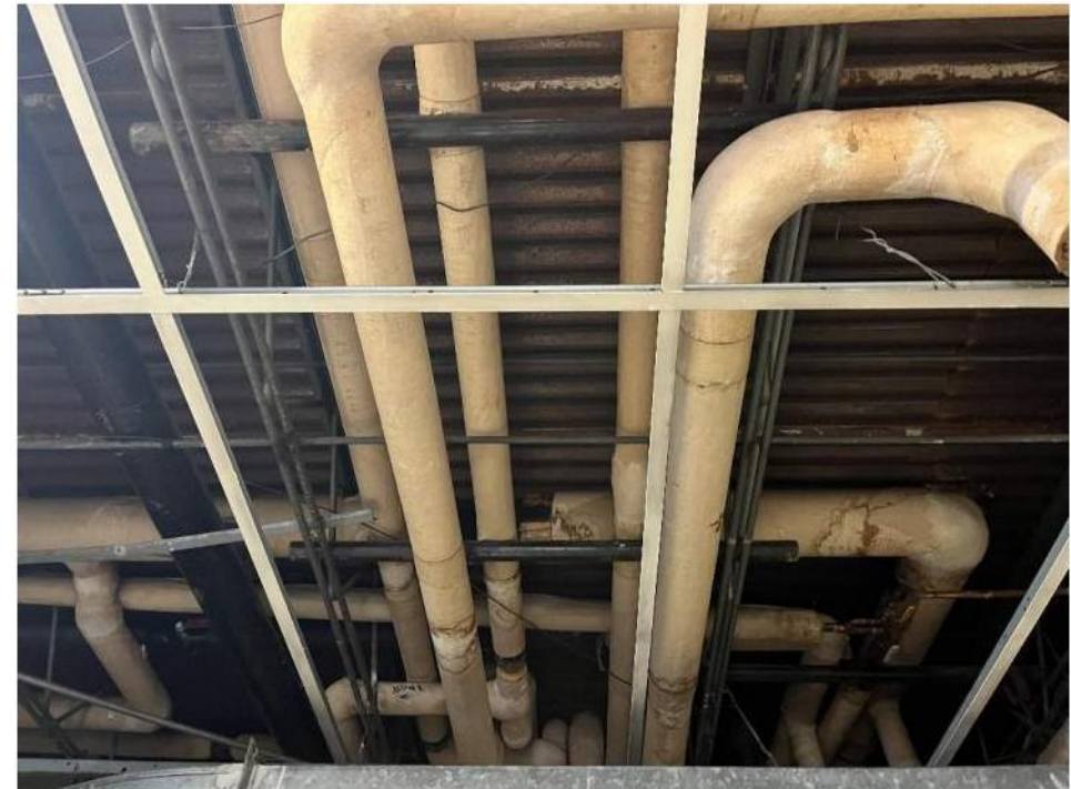
Deteriorating pipe insulation
