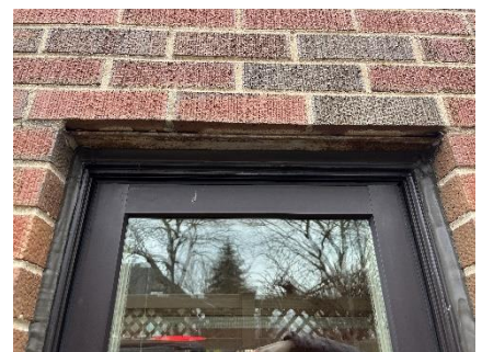
Corrosion at exterior steel lintels
