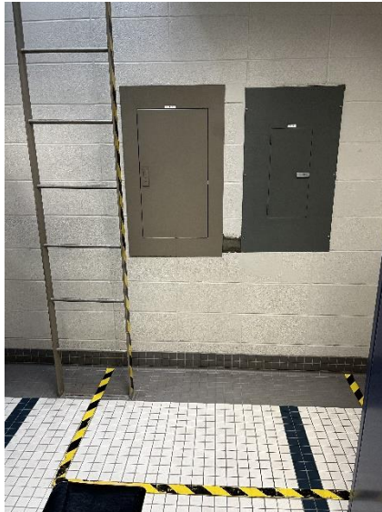
Roof access ladder projecting into circulation area
