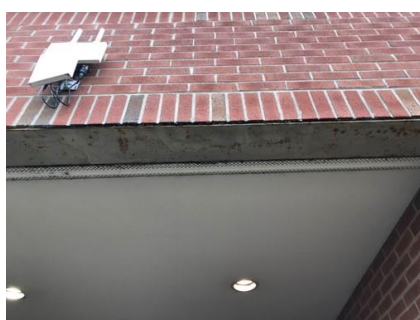
Surface corrosion at exterior lintel
