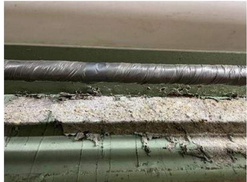
Deterioration at basement concrete wall
