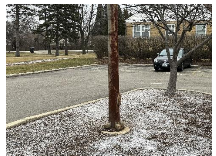
Significant corrosion at exterior site light poles
