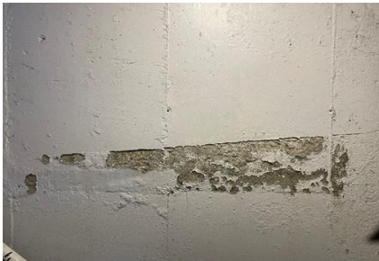
Efflorescence at basement stair
