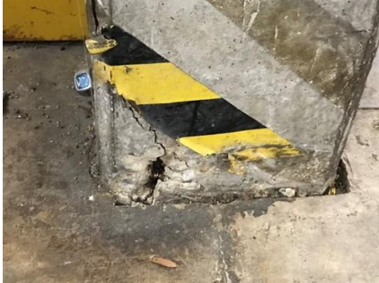
Column cracking at garage column
