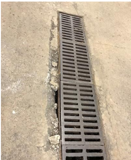
Concrete spalling at garage trench drain
