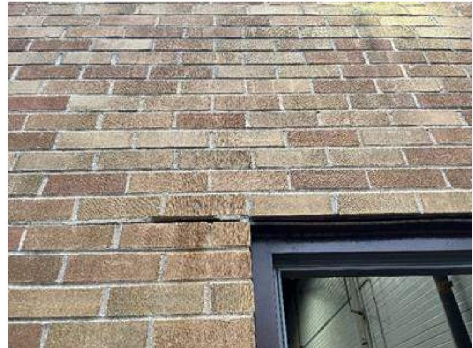
Step cracking and brick masonry displacement
