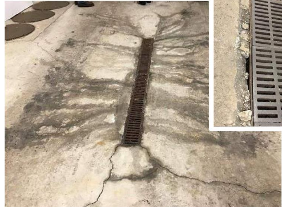
Concrete cracking at garage trench drain
