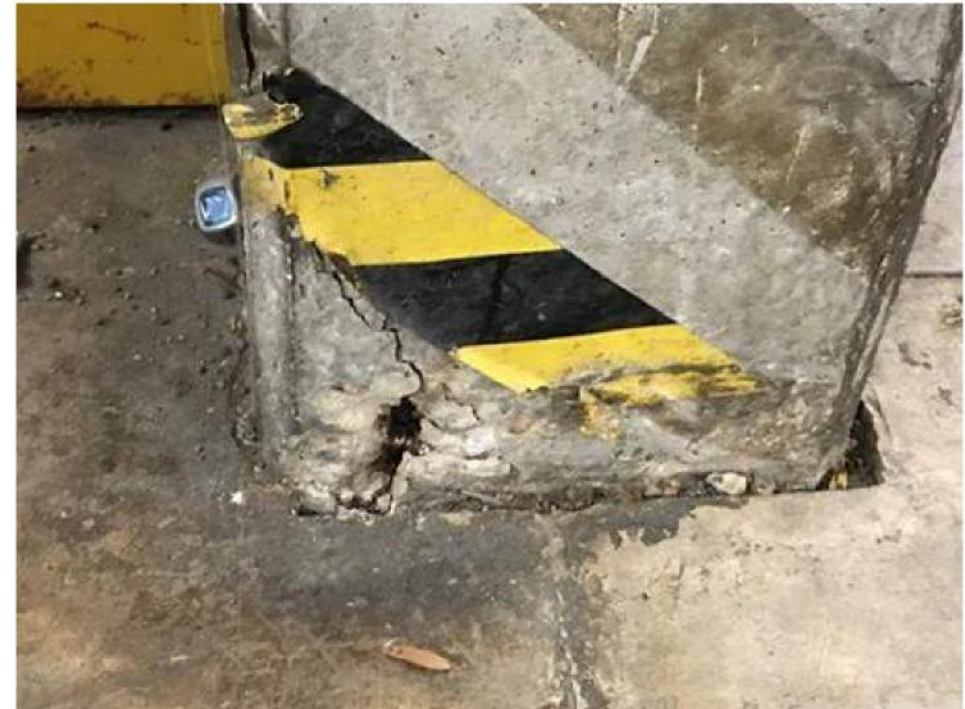
Column cracking at garage column
