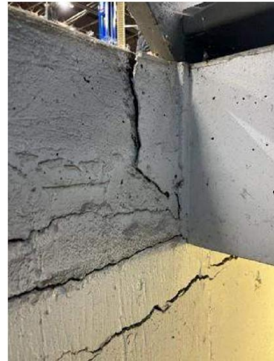
Significant concrete cracking at stair
