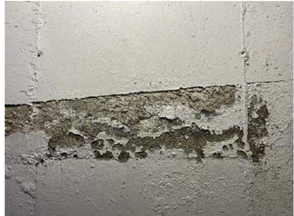
Efflorescence at basement stair
