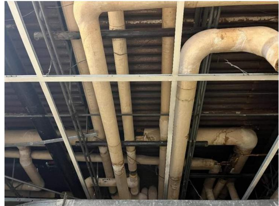
Deteriorating pipe insulation
