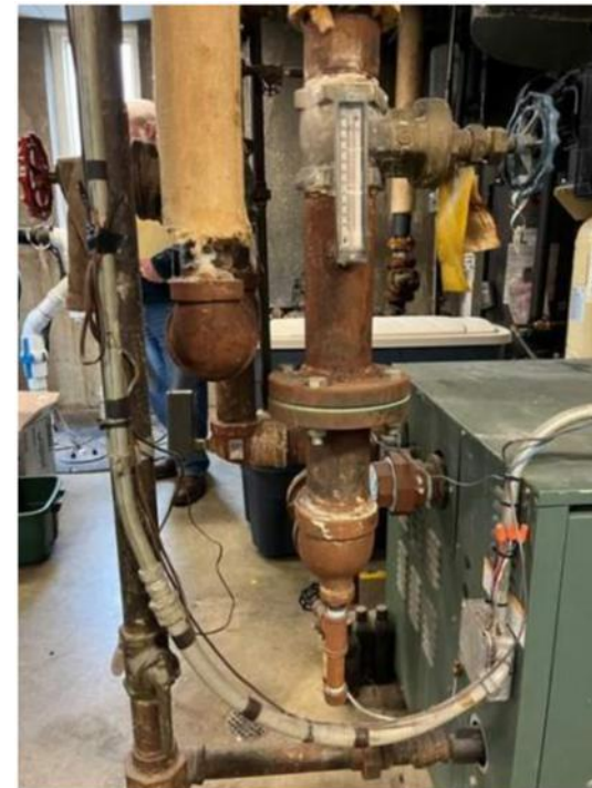
Significant corrosion on piping
