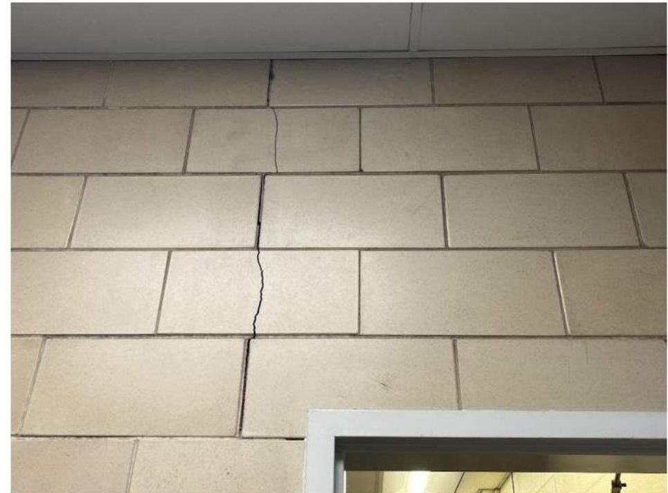
Cracking at interior masonry wall
