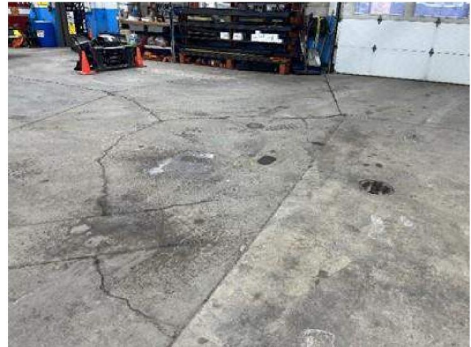
Concrete slab on grade cracking throughout
