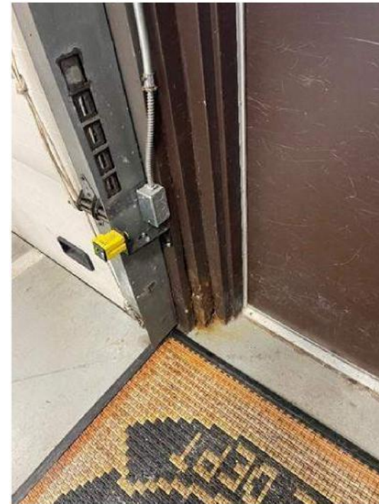
Significant corrosion at base of steel column in the Apparatus Bay
