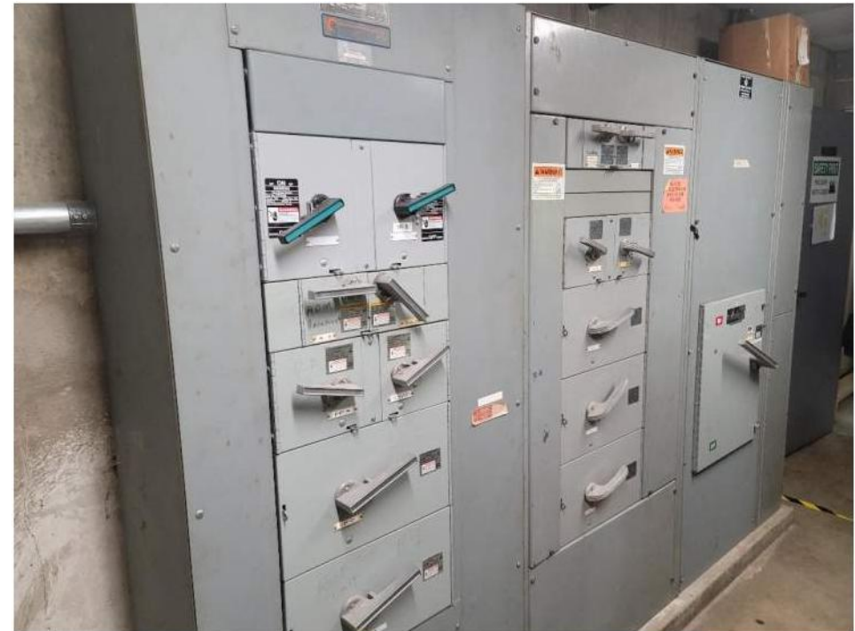
Original electrical service board
