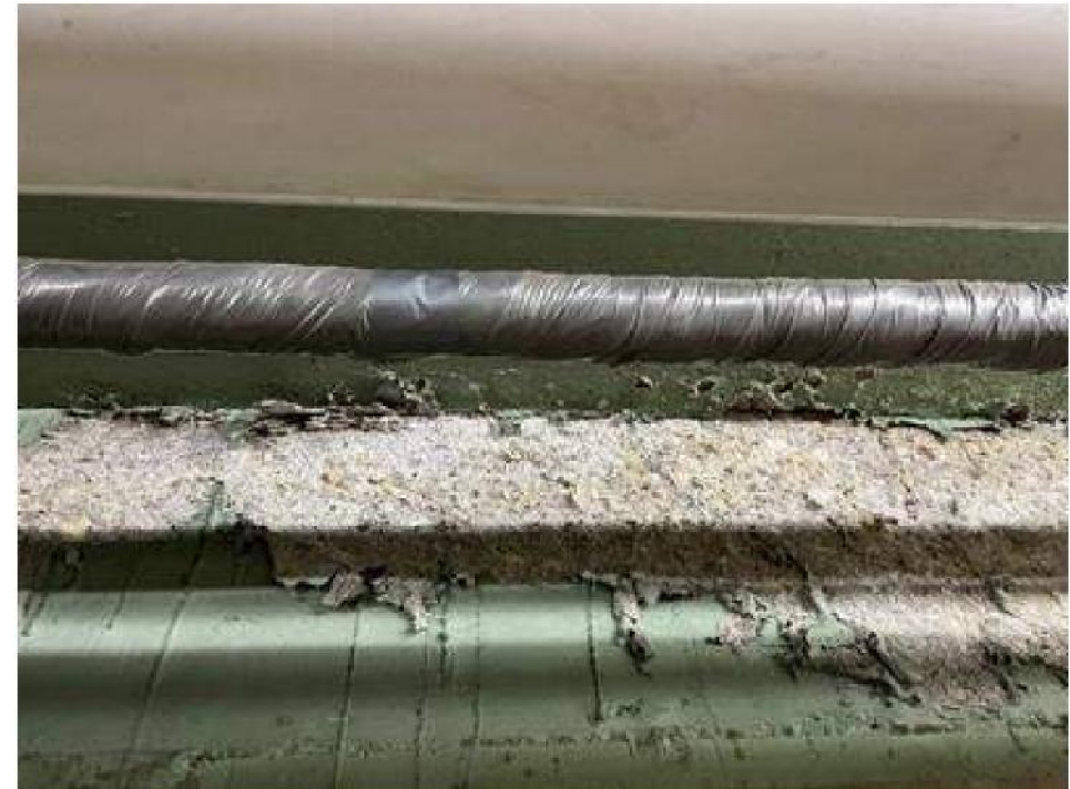
Deterioration at basement concrete wall
