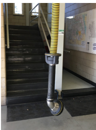
Stair between Apparatus and Staff Support floors
