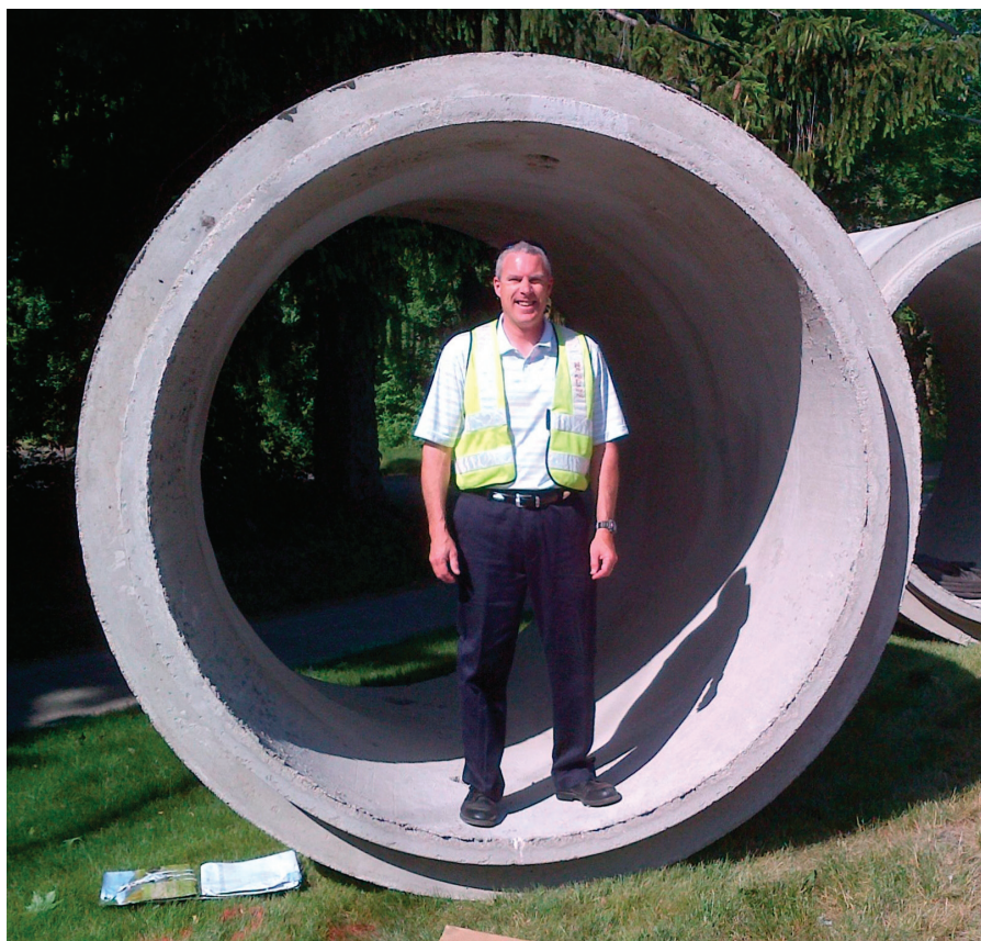
Northbrook's Village Engineer Paul Kendzior, 6-foot tall, stands in one of the 7-foot diameter sections of storm sewer that will soon be placed under Techny Road. The project is scheduled for completion in December 2013. For more information visit www.northbrook.il.us
