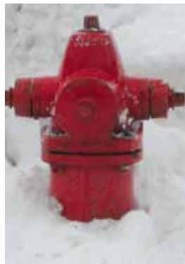
easy access. In addition to removing snow and debris covering the hydrant itself, it is recommended to clear a 3-foot area around the hydrant for easier access.
