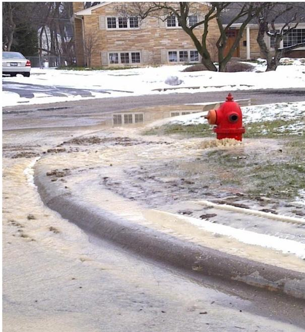
A third water main break was reported by the Police Department at 5:00 p.m. in front of 2018 Big Oak Lane. The break was on a 6-inch water main (1956) that is located in the parkway approximately 5-feet deep. Six homes were affected during the repair and were without water service from 7:30 p.m. to 9:45 p.m. A portion of the driveway apron for 2018 Big Oak Lane needed to be removed in order to complete the repairs to the water main.
