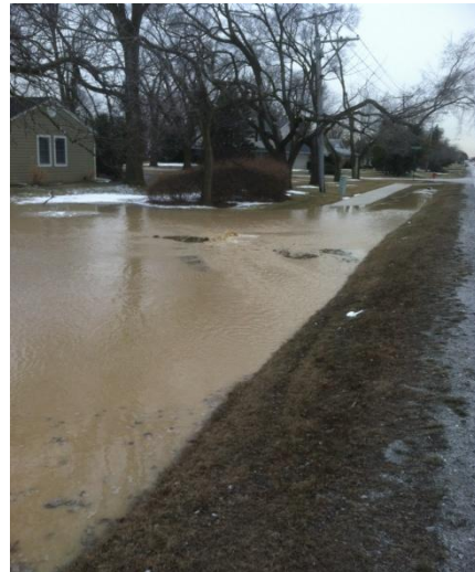
Pfingsten/Canterbury Road Water Main Break
