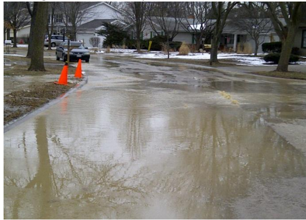
White Mountain Water Main Break
