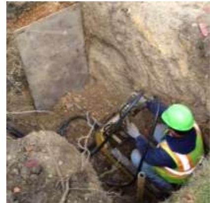
The photo depicts one of the contractor’s workers using a “push box” machine to install the water service lines underneath Crestwood Drive. This technology allows the service lines to be installed without excavating the roadway.
