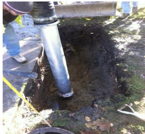
The sewer crew repaired a break in the sanitary sewer line in front of 2785 Appletree. Staff removed 7-feet of 8" broken clay pipe and replaced it with a 7-foot section of 8" PVC pipe. There were two services in the segment that were replaced. Staff used 6" PVC fittings to ensure a tight sealed connection on the two services.
