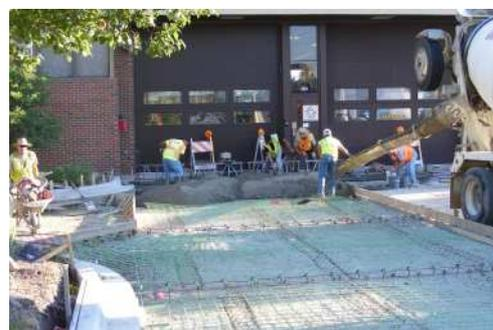
The concrete pavement panels at Catherine and Greenbriar have been removed and the granular sub-base has been placed. Concrete curb and gutter will be poured on Saturday, August 2. During the week of August 4, driveway aprons will be restored and the first layers of asphalt will be placed.
