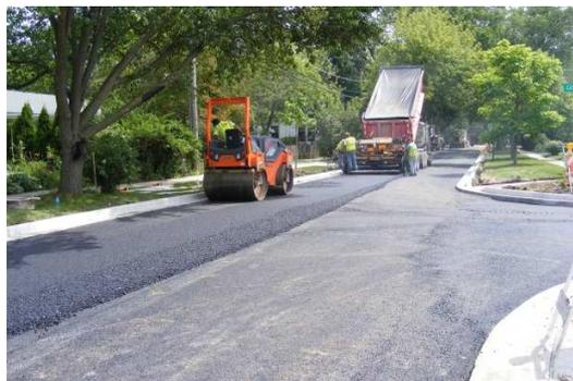
The reconstruction of Catherine and Greenbriar continued this week with the Village's contractor, A Lamp Concrete Contractors, installing the first layer of new asphalt and concrete curb and gutters (see photos).
