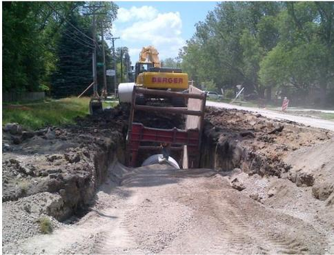
foot diameter pipe. Work completed this week included the installation of the 6-foot diameter storm sewer pipe from Glendale Avenue to Cargill Drive (see photo). It is anticipated that the intersection with Cargill Drive will be closed for the storm sewer installation on Wednesday and Thursday of next week. The Fire Department has been notified and plans to stage an engine at the south end of the street to respond to any emergencies that may occur on Cargill during the closure.
