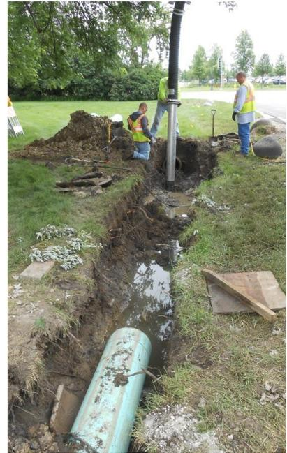
At approximately noon on June 14, the Northbrook Fire Department responded to the 1800 block of Old Willow Road for a reported natural gas line leak. Upon arrival, crews were advised that a 2" high pressure gas line was struck while crews were installing storm water pipes. Old Willow Road was shut down for approximately 2 hours while NICOR crews worked to shut down the leak and Fire Department crews stood by. Call-back personnel staffed reserve equipment during the incident.
