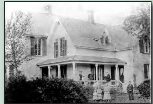
This large frame Sherman homestead, nestled beside the river on Shermer Road, was included in the Shermer land purchase. The site is now the home of the Village Presbyterian Church.
