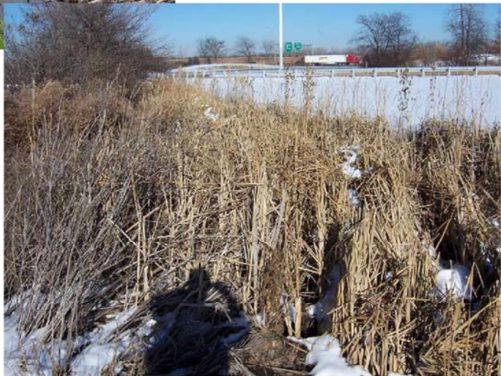
Outlet Channel is Heavily Vegetated
