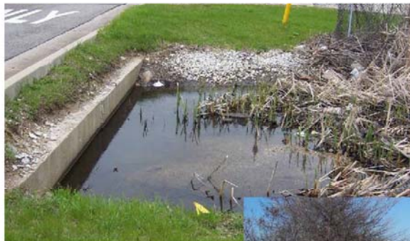
Outlet Box Culvert has Debris Impeding Conveyance
