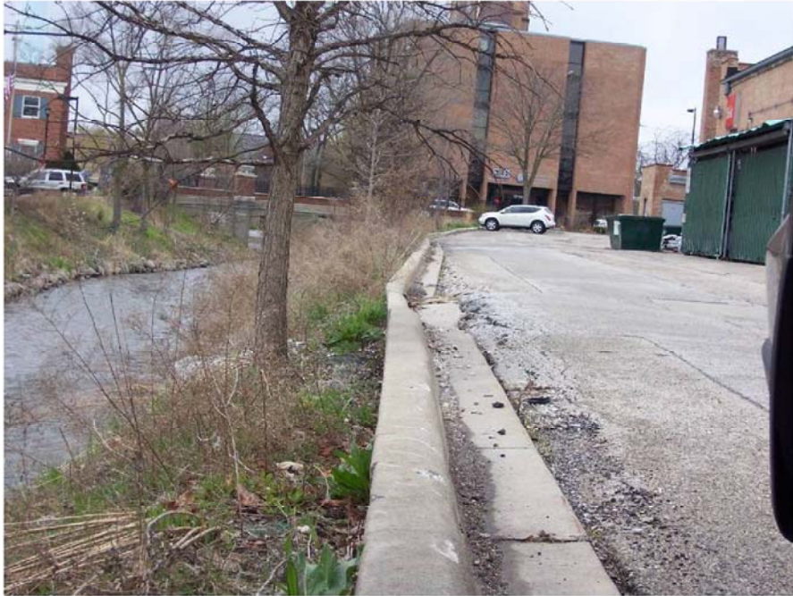
Curb Failure Looking Easterly
