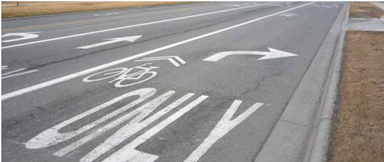
Shared lane markings and signs indicate that bicyclists should right in the left side of this right turn only lane.
