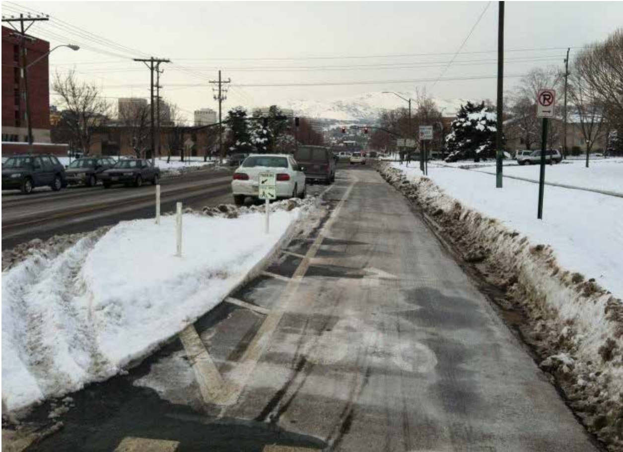
Protected cycletrack in Salt Lake City, UT after small truck plow snow removal. Photo Credit: Travis Jensen
