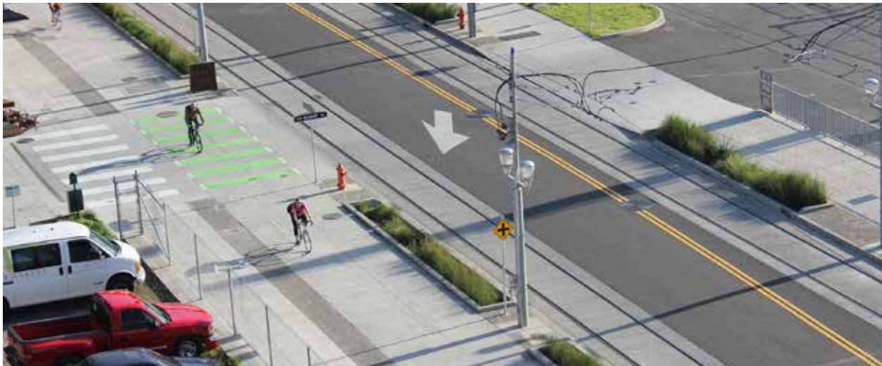
Intersection crossing markings can be used at signalized intersections or high volume minor street and driveway crossings, as illustrated above.
