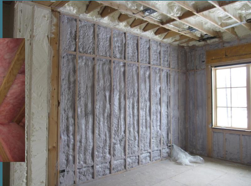
Note: To be considered within the conditioned space, ducts & pipes must have the full required R-Value between them and the exterior
