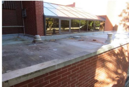
Central section modified bitumen roof
