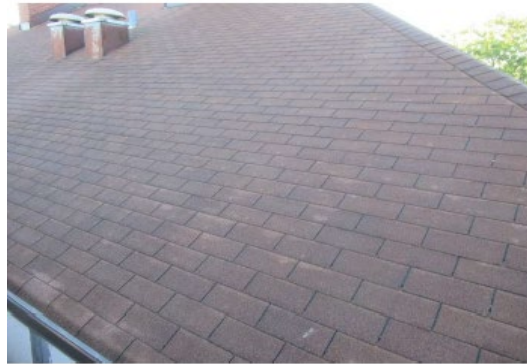
Shingles in fair condition with granule loss
