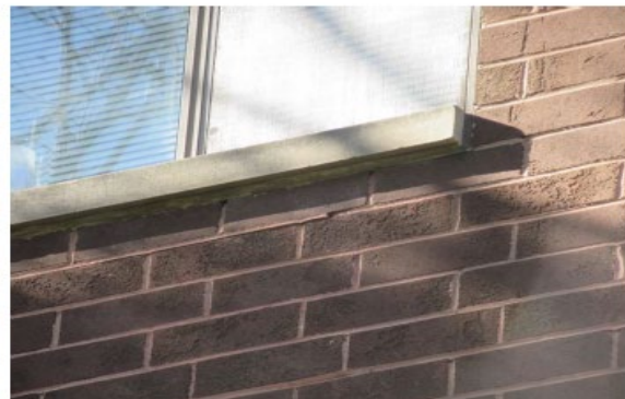
Mortar cracks and deterioration
