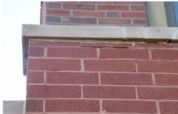
Mortar cracks and deterioration
