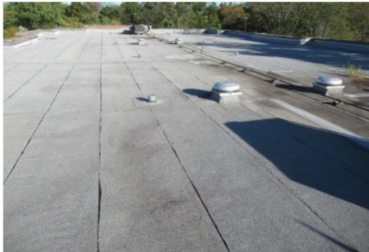
South wing modified bitumen roof
