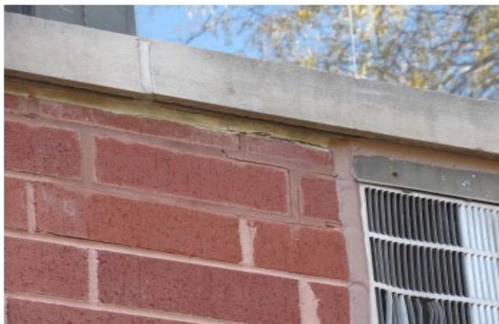
Isolated masonry and mortar cracks
